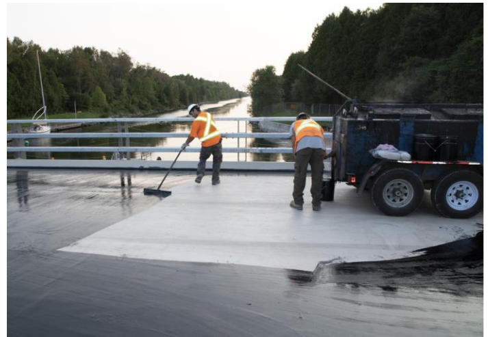
(b) Hand application of rubberized tack coat by using an oil-jacketed melter
