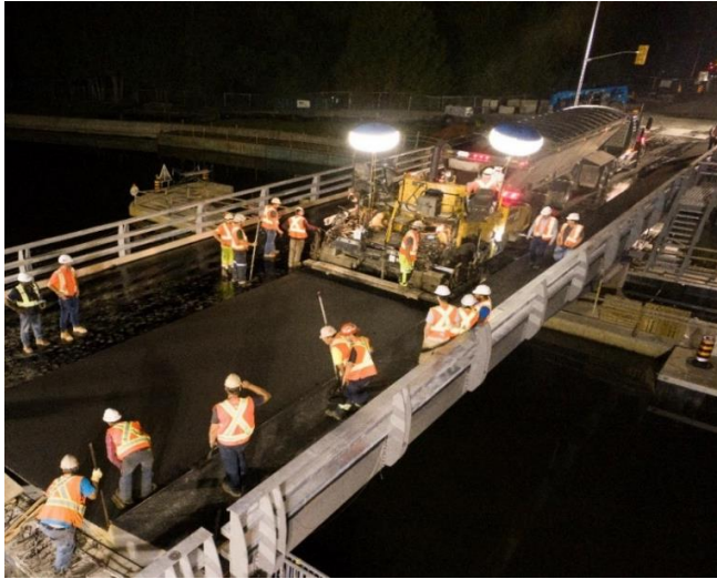
(a) Paving a low permeability asphalt mixture on an orthotropic steel bridge deck by using conventional paving equipment
