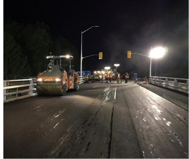
(b) Achieving targeted density after only three passes of 12-ton steel roller in static mode. The low permeability characteristics of the mix caused the release agent liquid used for compaction to stay on the surface
