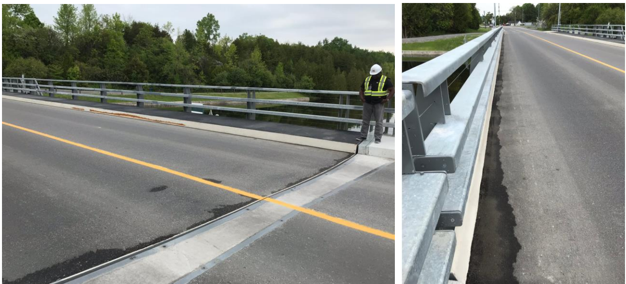
Figure 11. A Steel Swing-Bridge located in Southern Ontario after placement of Low Permeability Surface Mix (June 2018)
