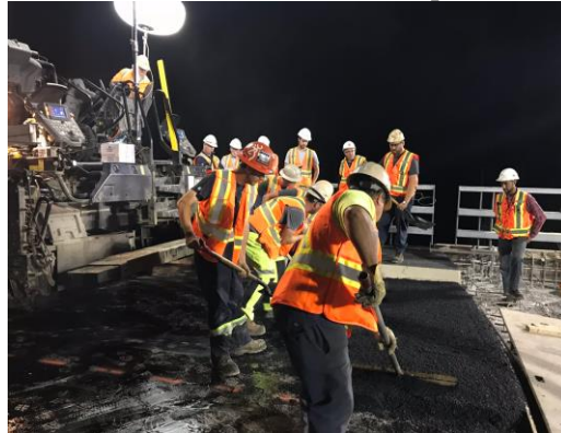
(d) Ease of handwork with sign of mix segregation
