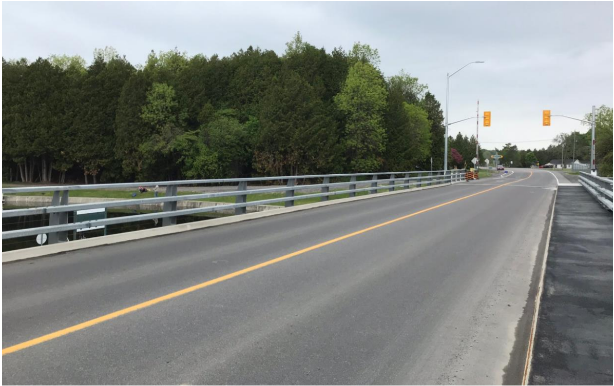
Figure 10. A Steel Swing-Bridge located in Southern Ontario after placement of Low Permeability Surface Mix (June 2018)
