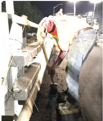
(c) No issues with using hand-roller to compact around the hard-to-reach areas
