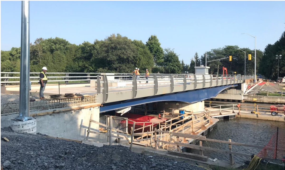
Figure 6. An Orthotropic Steel Swing Bridge located in Southern Ontario prior to placement of Low Permeability Surface Mix (August 2018).
